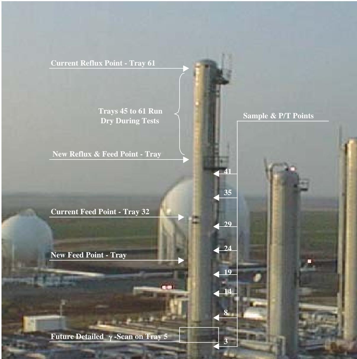
**Figure 6 Photograph of 4P Tower Showing Additional Features**
