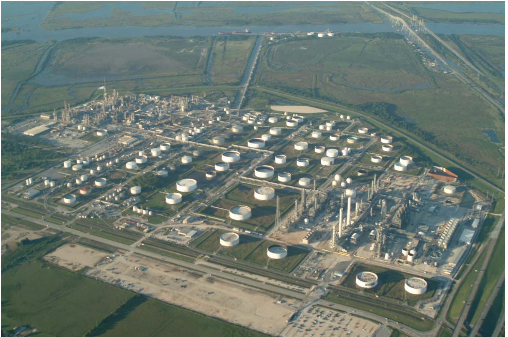
Figure 2 BASF FINA Petrochemicals LP(Naphtha Cracker) and Sabina Petrochemicals LLC
